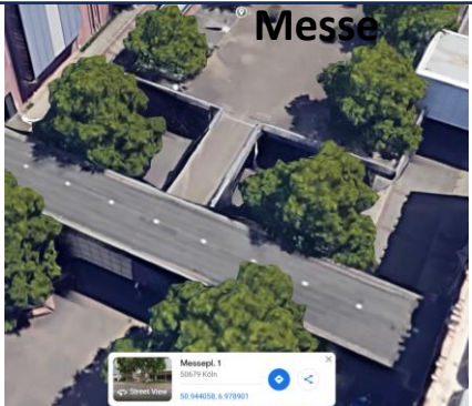
Parking garage of the Köln Messe
